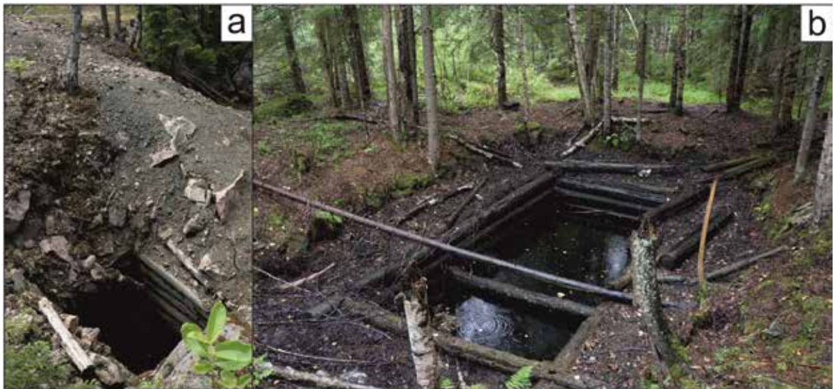
Figure 1. Photographs of the flooded eastern (a) and western (b) mines in the Beck mine field, captured by the authors during field campaigns in 2021 and 2022.
