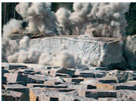
Figure 4. Ladozhskoe deposit on the Karelian Isthmus (Leningrad region). Splitting up of primary monolith using blast-hole technique.
